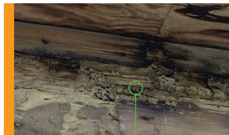
Termite Damage
